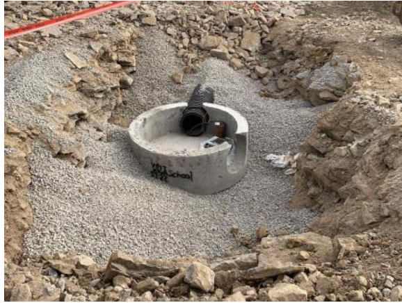
Storm manhole installation near future JV softball field (11/03/2021)
