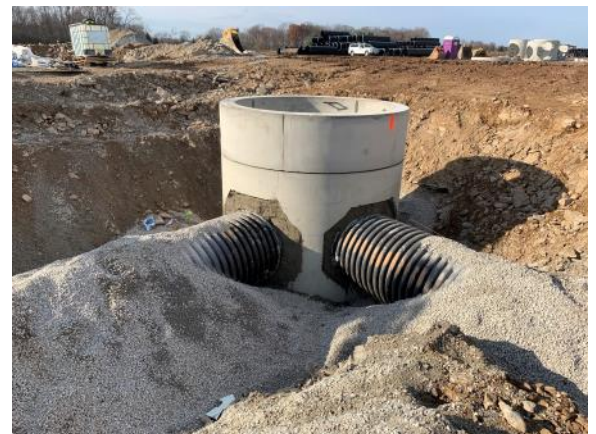
10' wide storm manhole under future road by tennis courts (11/16/2021)
