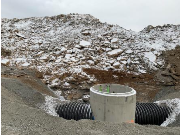
Installation of storm manhole near football practice fields (11/29/2021)
