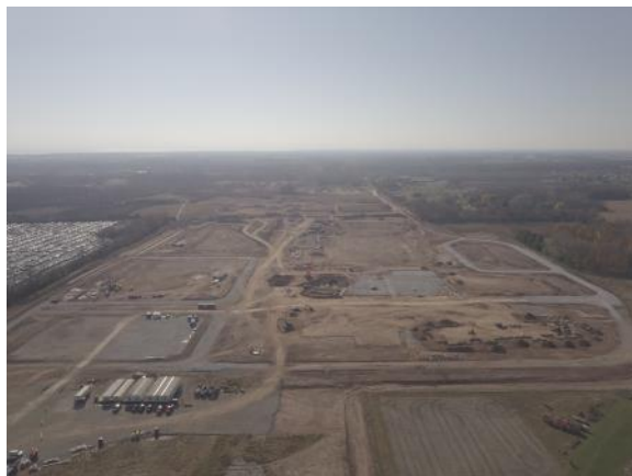
Overall view of site looking South (11/08/2021)
